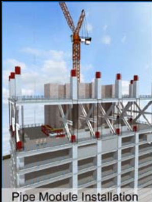
Pipe Module Installation
