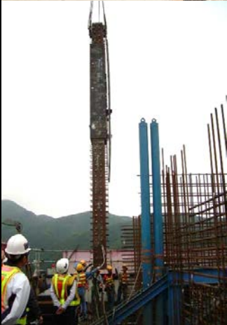
Steel Outrigger and Rebars
