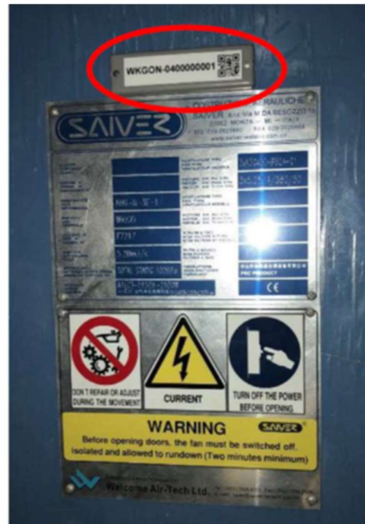
Figure 7-4 RFID Tag for AHU (Next to the Nameplate)
