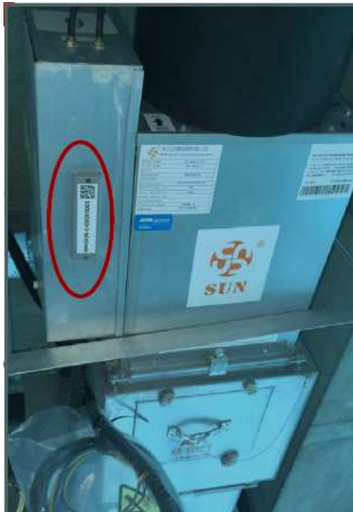
Figure 7-3 RFID Tag for VAV Box
