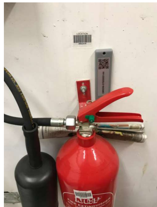
Figure 7-10 RFID Tag Next to the Bracket of Fire Extinguisher
