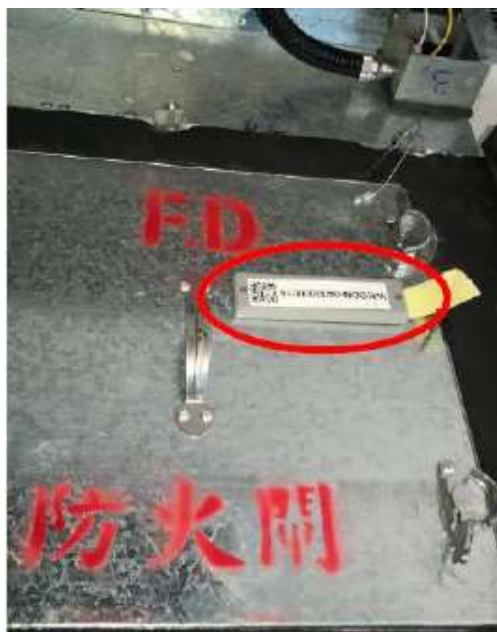
Figure 7-5 RFID Tag for Fire Dampers
