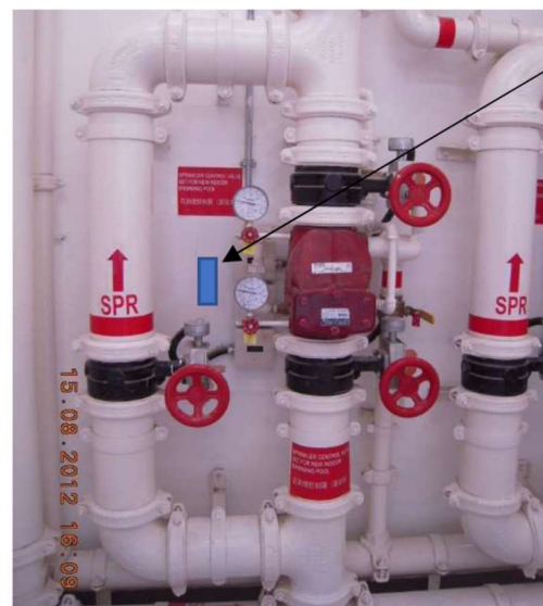
Figure 7-6 RFID Tag for Control Valve Set
