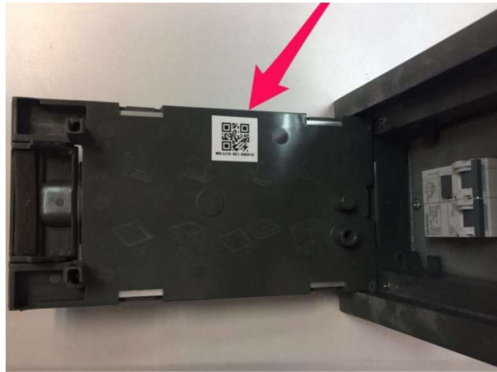
Figure 7-7 Zone Tag at Floor Box
