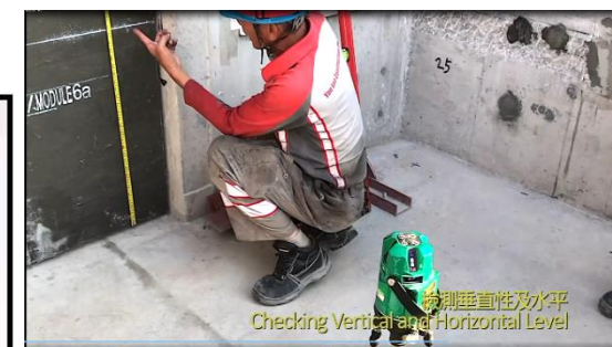
Figure 9.21: Checking vertical and horizontal level (Source: Yau Lee Construction Company Limited)
