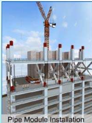
Pipe Module Installation
