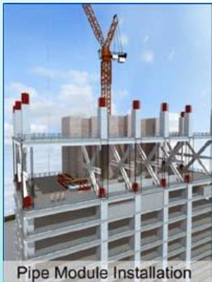
Pipe Module Installation
