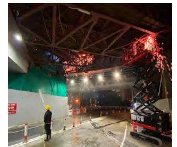
Implementation of steel truss removal
