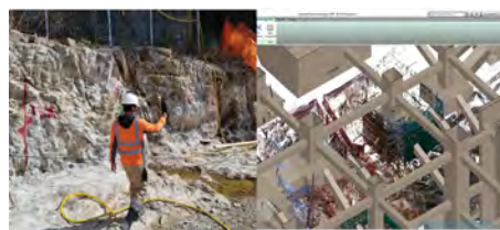
Surveying with 3D handheld scanner seamlessly integrating site condition into the BIM model. Image Courtesy of Architectural Services Department, HKSAR and Shui On Joint Venture and WSP Hong Kong Limited
