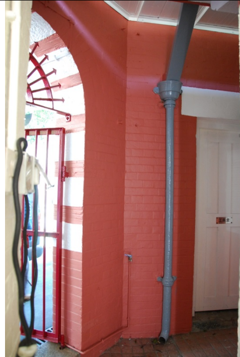
Figure 2: Rainwater Downpipe at Former Peak School. (Source: ARTitects Limited)
