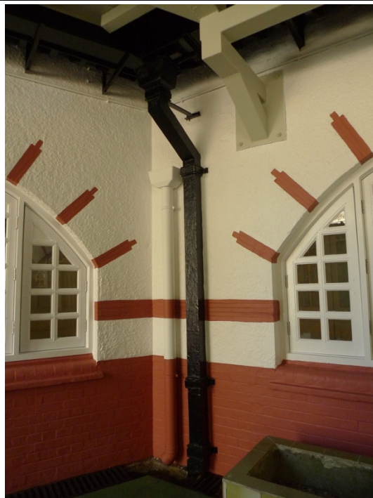
Figure 12: Rainwater Downpipe at Former Peak School. (Source: ARTitects Limited)
