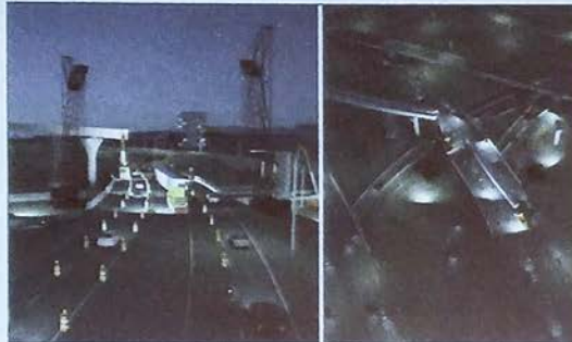
Workers on boom lifts, girder delivered in median
