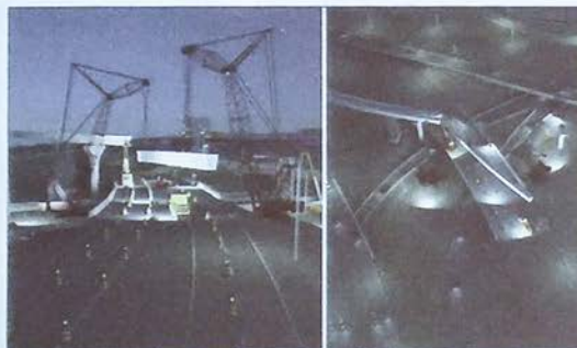
Girder lifted from delivery vehicle
