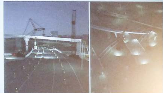
Girder lowered into final position Maximum 8' into ground and temporary being lowered moved for 28.5' N/S
