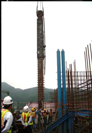
Steel Outrigger and Rebars
