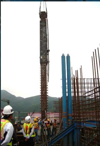
Steel Outrigger and Rebars
