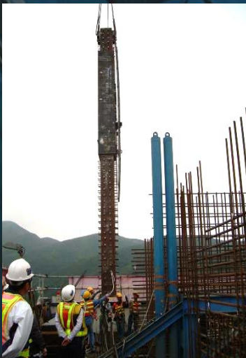
Steel Outrigger and Rebars
