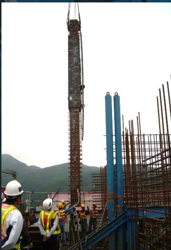
Steel Outrigger and Rebars
