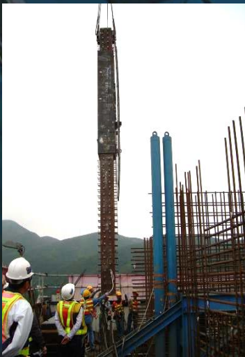
Steel Outrigger and Rebars
