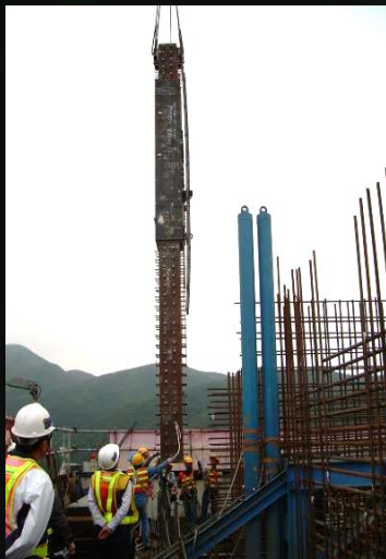
Steel Outrigger and Rebars
